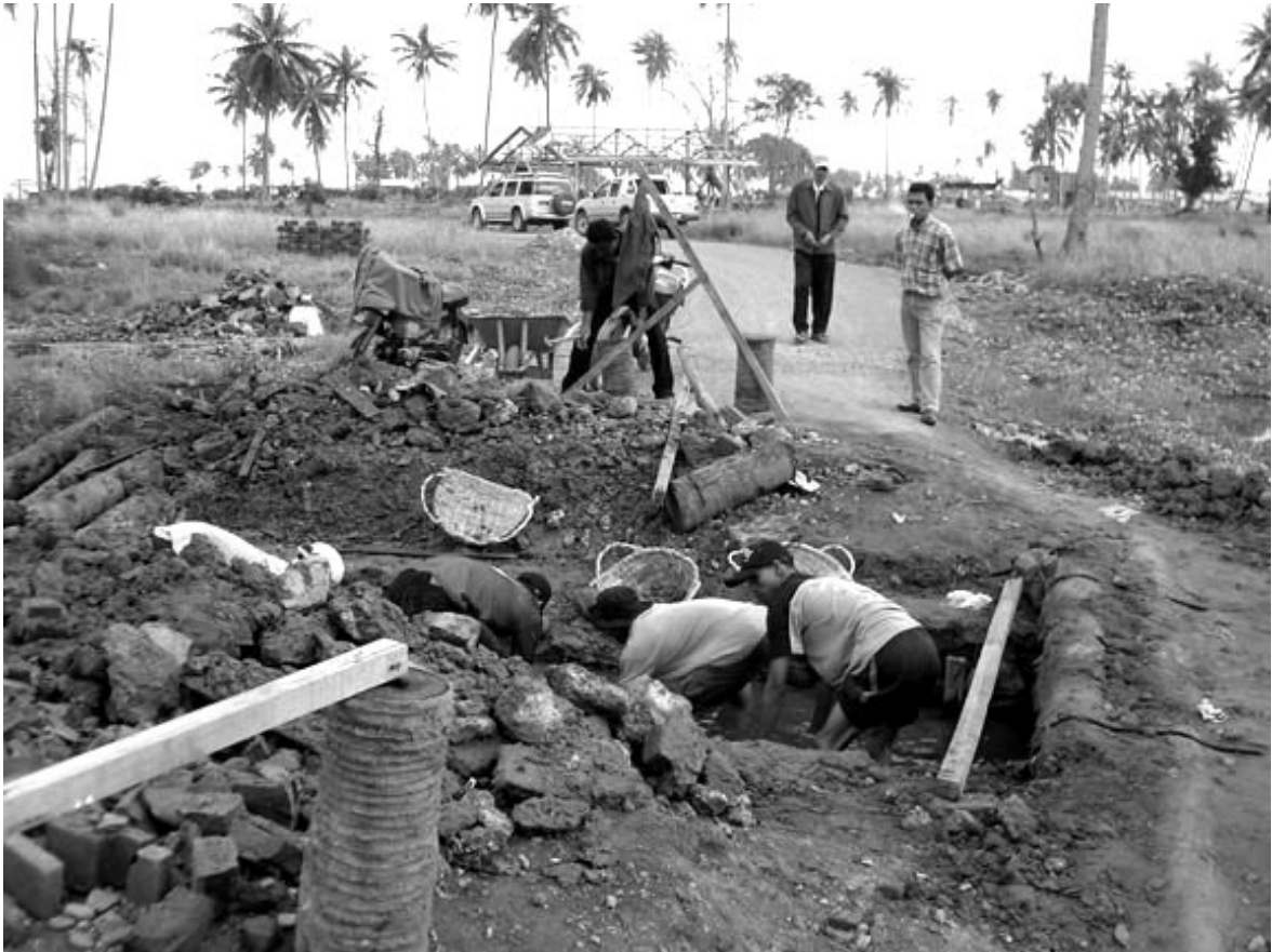
Recovery work after the tsunami in Banda Aceh, Indonesia
