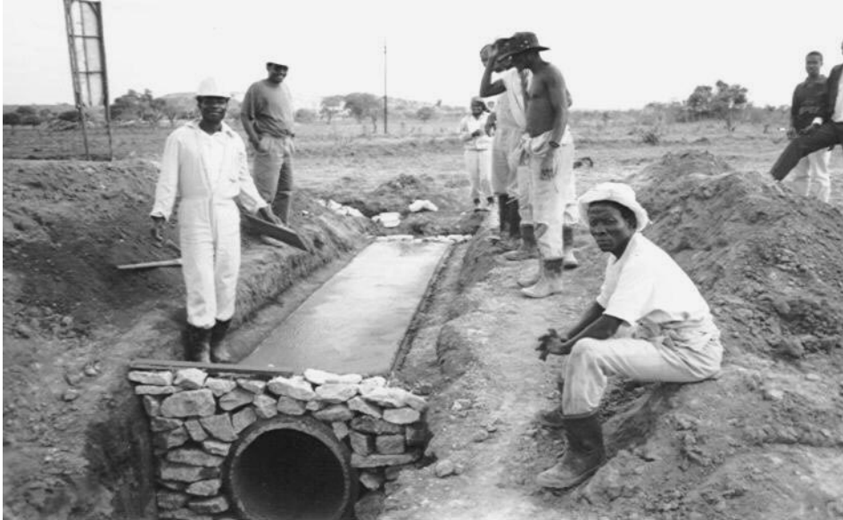
Laying of culvert pipe in Mozambique
