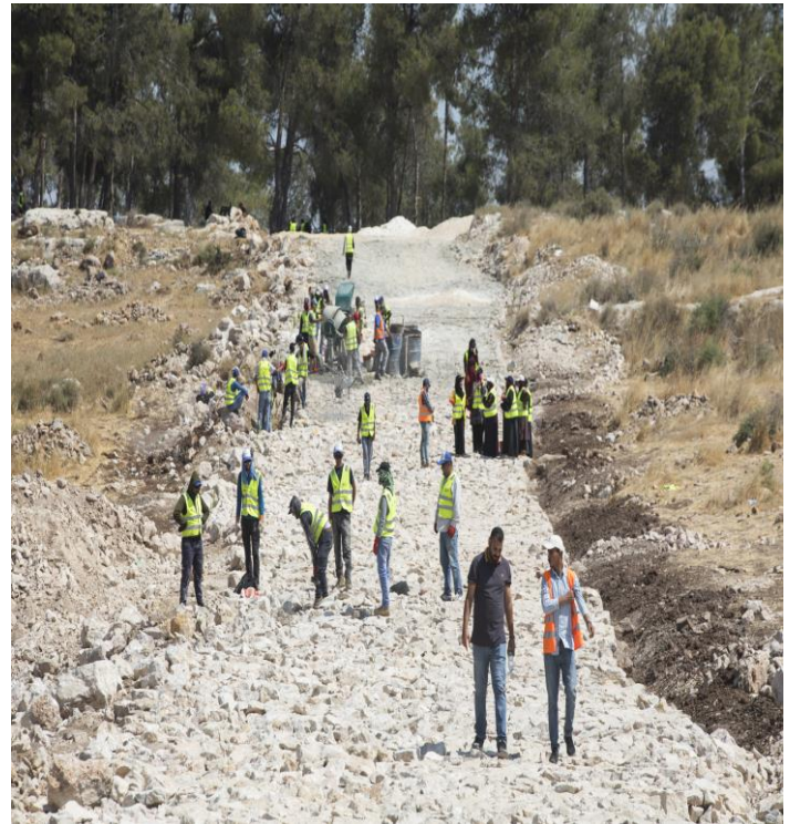
Group of workers doing a stone pavement for a rural road in Rabeyat alKoora Municipality - Irbid Governorate
