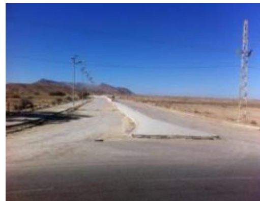
Ring road bypassing Gafsa (15 km 2x2 lane)
