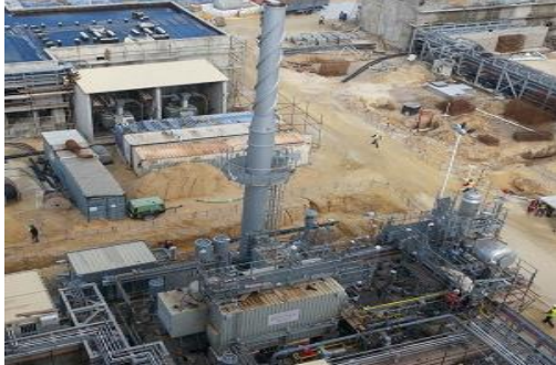
Power Station Sousse C
