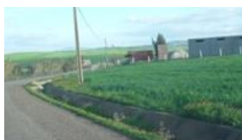
PNRR-2 Sample Road in Khmeissat
