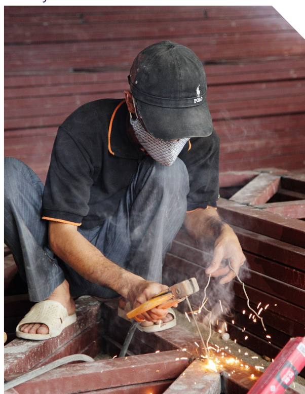
An informal labourer welding metal at a construction site. © ILO
