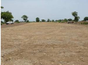
This picture shows a section of a large size dam that apparently was compacted using a 200kg non-vibrating roller. It is obvious that layer of fill material is not really compacted to the required density (too many voids between the soil particles).
