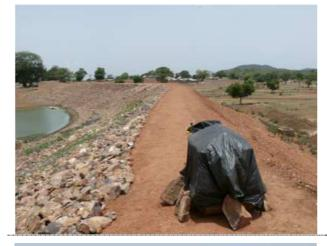
On this dam (practical training demonstration site) the work has been completed to good quality and apparently compaction was done to satisfaction. (compaction equipment covered with black plastic sheet)
