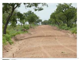
Problems with setting out and controlling horizontal and vertical alignments. Most standard setting out tools for LI work activities are missing on site. The formation material is not compacted.
