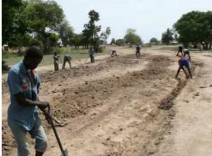
No setting proper setting out of drainage activities i) to ensure that drain is excavated to the correct size and gradient, and ii) to ensure that the ditch material is heaped along the centre line of the road to be later used to form the camber.
