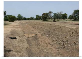
Drain material is heaped along the shoulder-line instead of along the centre-line. The template used has the wrong shape as it is of the full drain shape including fore and back slopes. It cannot be used for ditching and sloping, but only for backsloping.
