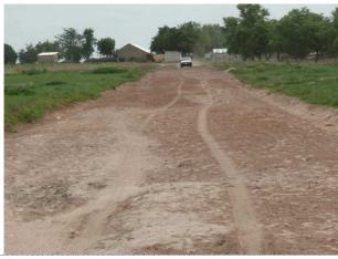
The result of the above work practice is a 'flat' road without any camber crossfall, poor drainage, uncontrolled vertical and horizontal alignments and uncompacted formation / gravel course.
