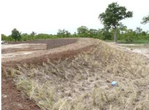
Dam work in general is of good quality apart from insufficient and uncontrolled compaction of fill material.
