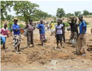
The right tools for the job are required for productive LI work. These labourers are using mattocks to spread fill material. Spreaders would be much more effective and would allow for a more uniform layer. To control the layer uniformity and thickness appropriate levels should be established and marked with level pegs and strings as well as checking with straight edges to detect depressions or areas with too much material.
