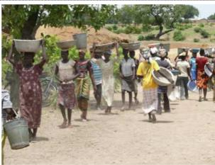
These ladies are head-carrying hundreds of tons of fill material using their own head-pans or buckets. Each of them has a different shape and size. The task given is however a group task for over 160 labourers. Is this a fair and controllable arrangement?
