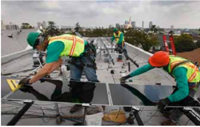
Installation of solar panels
