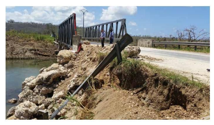
missed the northern provinces of Torba and Sanma, the associated rain caused flooding damage to culvert crossings, road pavements, and aerodromes in these two provinces.<sup>38</sup>
