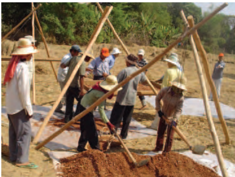
Construction workers in Battambang, Cambodia, sift laterite for use in building roads. Photo: ILO/Van Samsan, March 2007.
