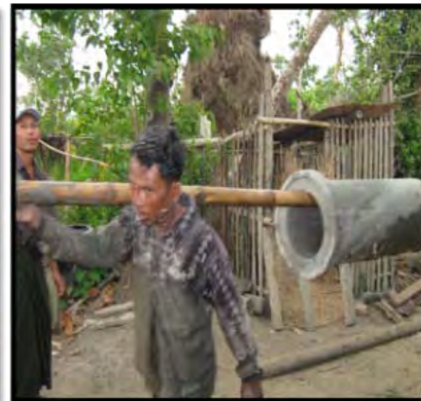
3. Transporting concrete pipe
