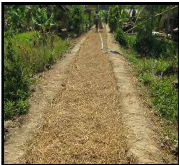
10. Curing of concrete
