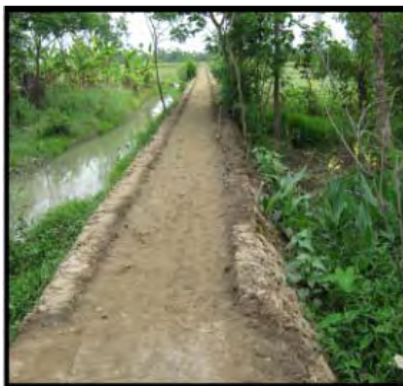
5. After compaction of base
