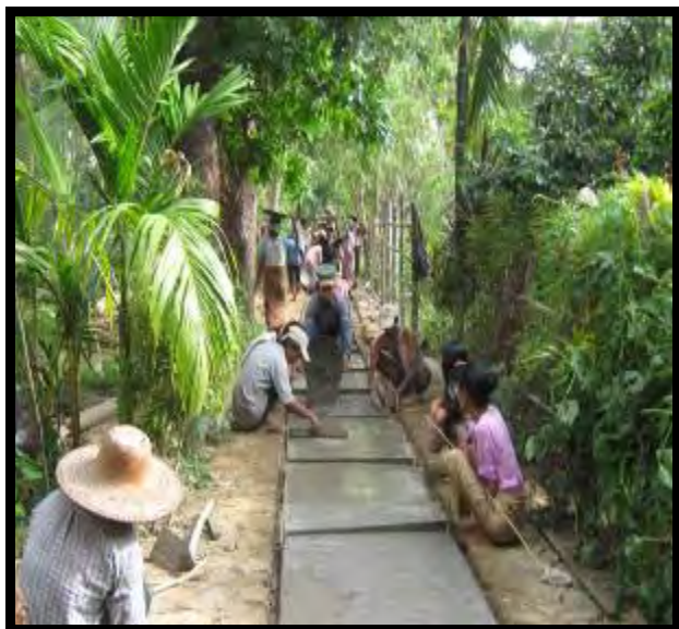
7. Pouring of concrete
