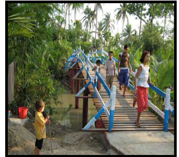
21. After Construction of Bridge
