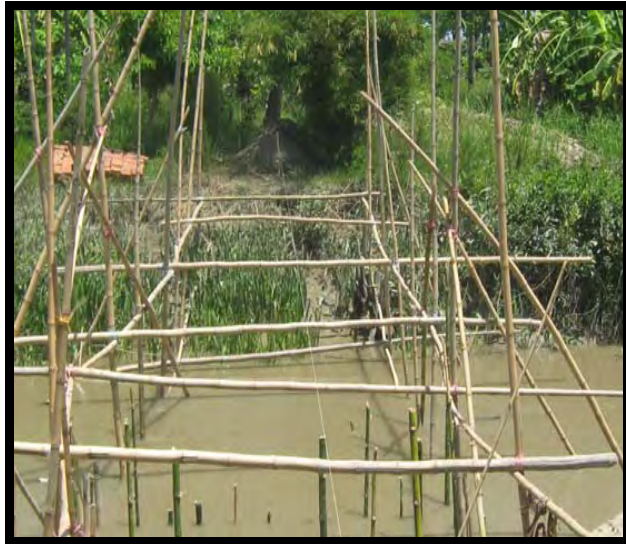
19. Scaffolding at bridge site
