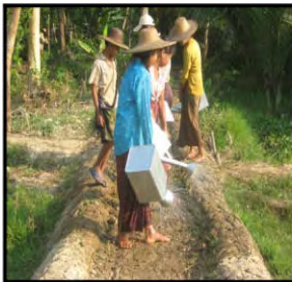
2. Spraying of water before compaction
