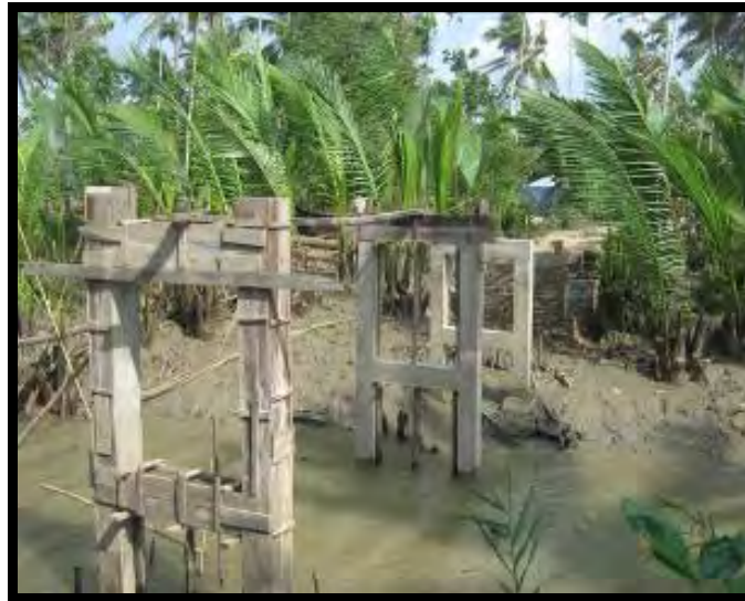
20. Piers of the Bridge
