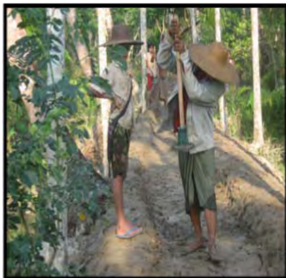
4. Compaction of footpath
