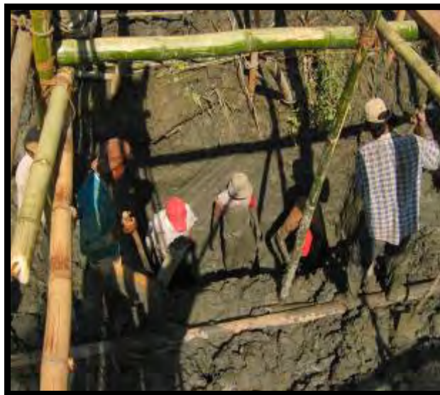
17. Foundation of piers of Bridge
