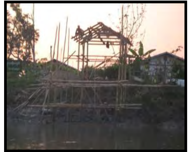
15. During Construction of Jetty
