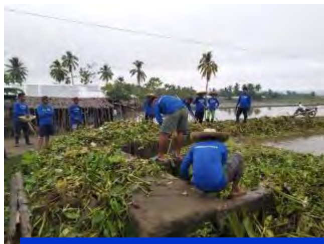
CEEP workers conduct flood-control activities.
