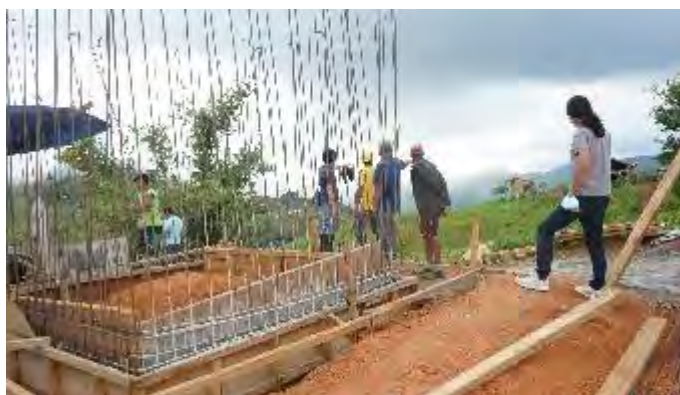
Water tank construction in Renti, N. Upi, Maguindanao.
