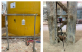
1. Profile in-situ environmental conditions at worksite
