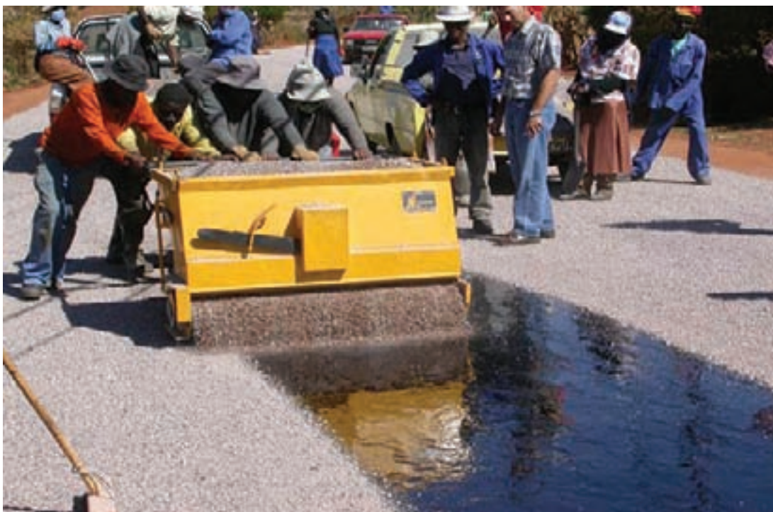
Road construction through labour-intensive methods
